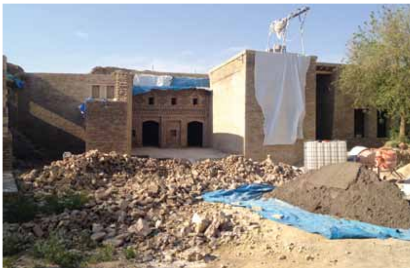
Work is now under way to restore and reconstruct the elegant 19th-century mansions and palaces that cover much of the citadel. These residences of the wealthy fell into ruin during the last several decades.
